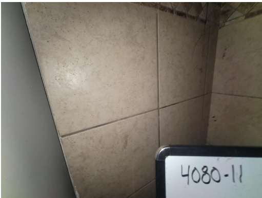
4080-11 Ceramic Tile/Grout/Mortar Typical Interior Bathroom
