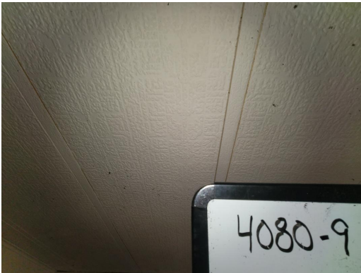
4080-9 Ceiling Paneling Typical Interior
